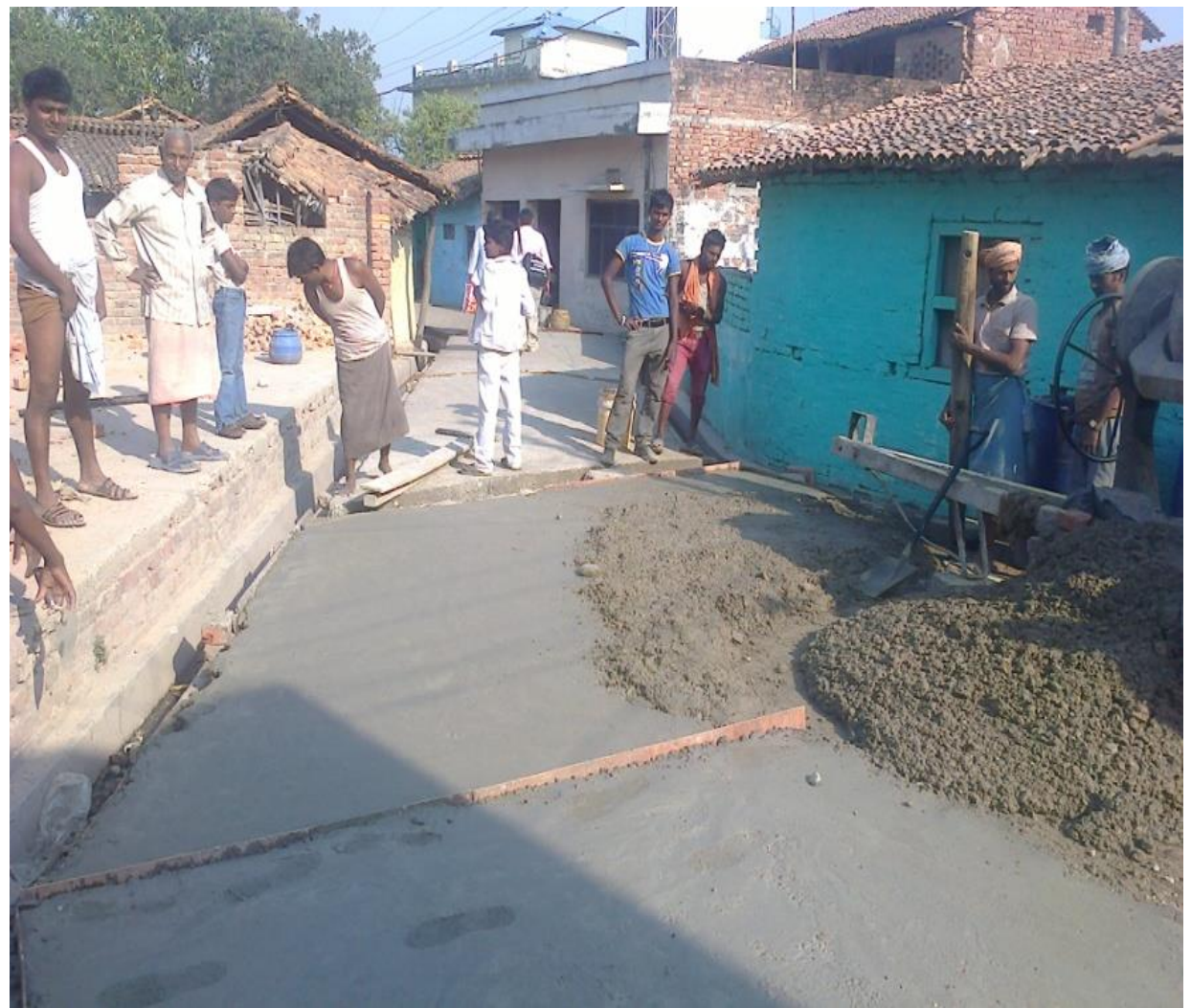
Road PCC Work With Side Drain at Ward no. 7, Near Dusaad Kutti Total Exp. 535771.66 (30% User's Committee contribution Included)
